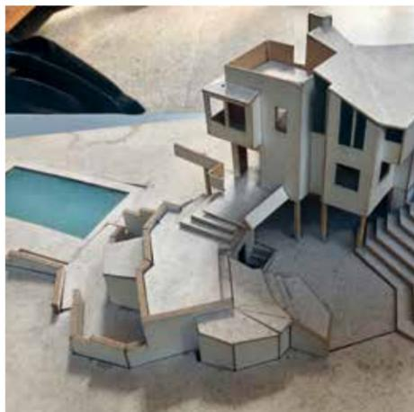
*classic roof. The choice of timber and pilings and their decoupling from the natural soil ensure that its structures and terraces have been perfectly preserved for more than three decades.*
